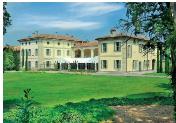
Villa Torri (Fonte www.villatorrimorpurgo.com )
